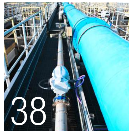
Tai Po Sewage Treatment Works is upgrading its aeration tanks with over 100 AVK Series 76 butterfly valves.
