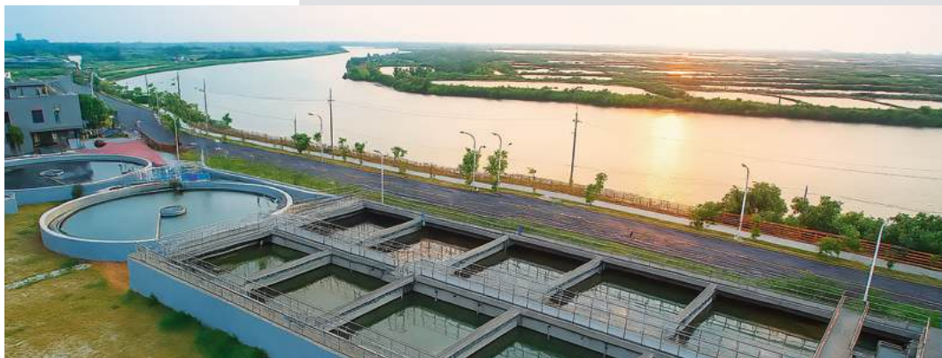
Aerial view of Annan Water Resources Centre
